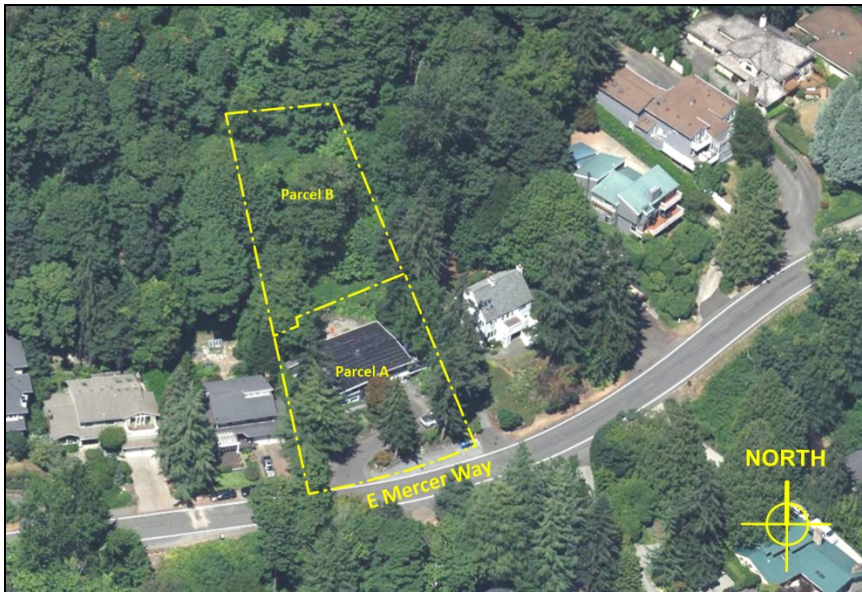
Plate 1: An aerial view of the project site.
